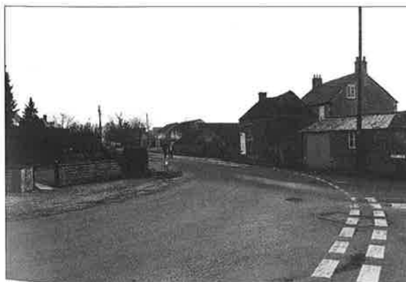
Fig 4: The Kent End junction with Fore Street. The view shows the bend at this point, note the width of the junction.
