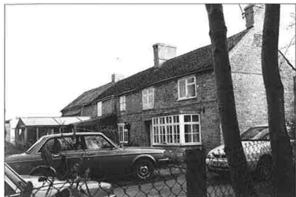
Fig 5: No 5 on the east side of Thames Walk, taken from the back.
