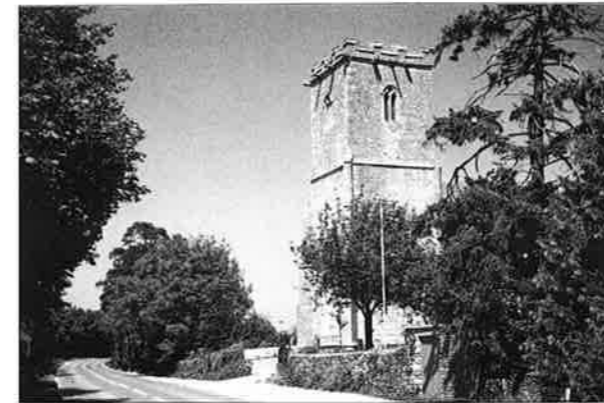
Fig 8: The presence of the Church of The Holy Cross as approached from the south on the B4696
