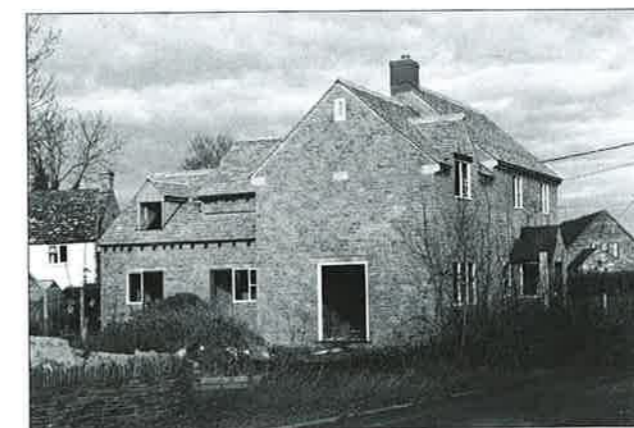
New house under construction at Rixon Gate
