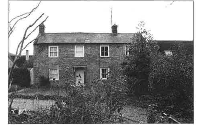
Fig 12: The Old Police House. The position of the stack and porch betray the added bay at the right.
