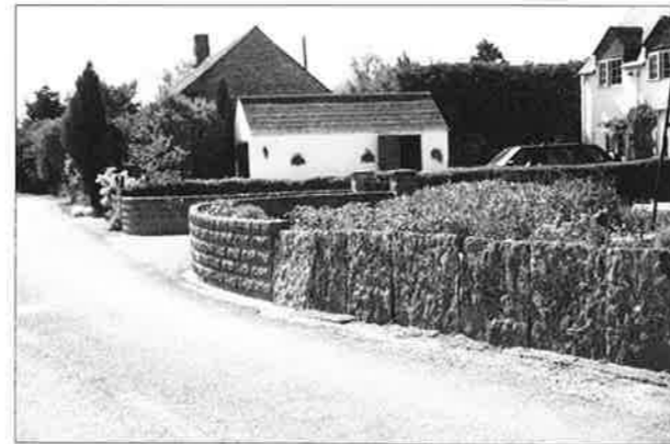
Fig 4: Orthostatic boundary wall along The Derry adjacent to modern walling.
