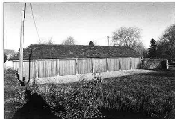
Fig 4: Farmstore building at Church Farm.
