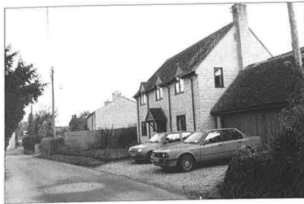
Fig 1: The absence of a frontage boundary wall is starkly obvious where missing from a recent infill house. Other lessons from this building can be learnt - the inappropriateness of the artificial stone, due to its blue colour quite unlike the local stone; the lack of roof overhang at eaves; the size of house relative plot, and lack of front garden wall/planting.
