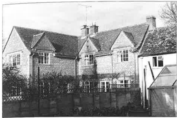
Fig 4: Nos 3 and 4 on the west side of the Thames Walk, taken from the back.
