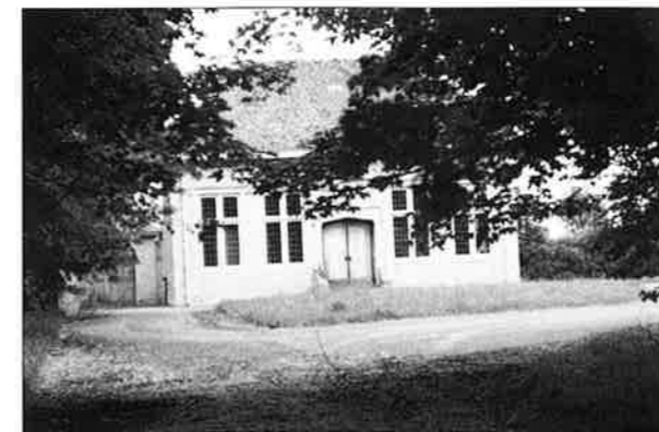
Fig 10: The pumping station.
