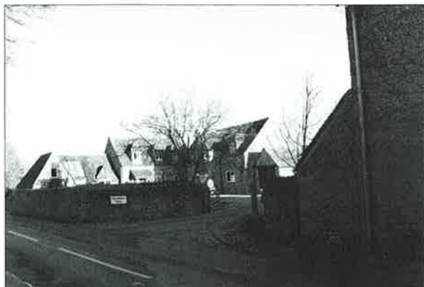
Fig 1: The converted barns at Manor Farm. The farmhouse is in the foreground
