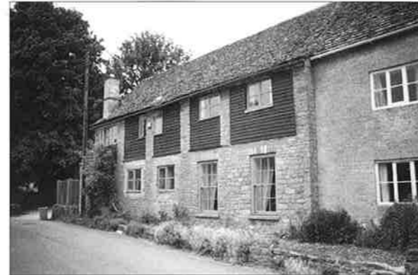
Fig 10: The Tannery and Cleveland House are semi-detached. There is only a short stretch of road visible before the bend.
