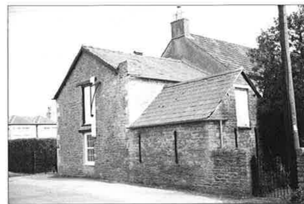
Fig 10: No.23 with hoist detail
