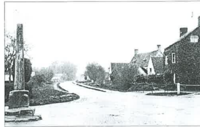
High Road Cross. In 1958 this cross adjacent to the White Hart was relocated to avoid danger of damage by vehicles.
