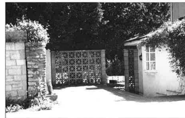
Fig 12: Replacement walling inappropriate to conservation area
