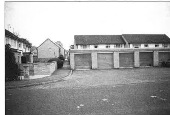
Fig 9: Communal garages at Harris Road.
