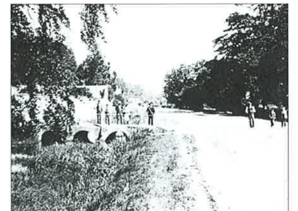
Fig1: Derry Bridge in High Road, looking north at the turn of the century.
