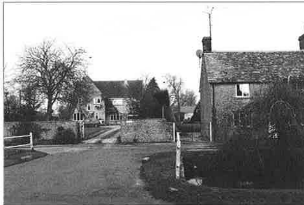
Fig 2: Glebe House & No 9 Church Lane, showing long driveway to the former, by contrast with the latter's frontage straight onto lane (note obtrusive satellite dish location). Glebe House, a rather suburban 1950s house higher and larger in plan than its neighbours along Church Lane, well separated by being set-back 30m behind a low wall & screen of shrubs. This distance reduces adverse impact that this house would otherwise have on its neighbours. Extensions have resulted in a building constructed of three clearly different types of reconstituted stone. Although efforts have been made to match the general colour, it is a prime example of the incongruity of artificial stone, and the problems of development out of character with this corner of the village.
