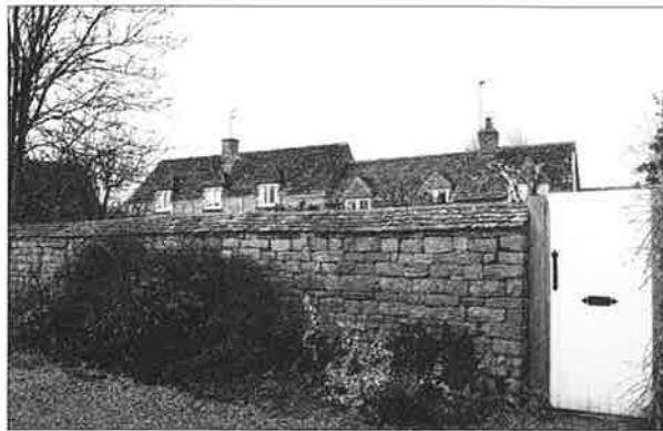
Fig 4: No 1 and No 2, Wall Cottage.
