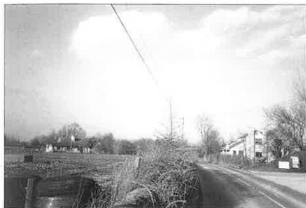
Fig 4: View north, with workshops on the right.
