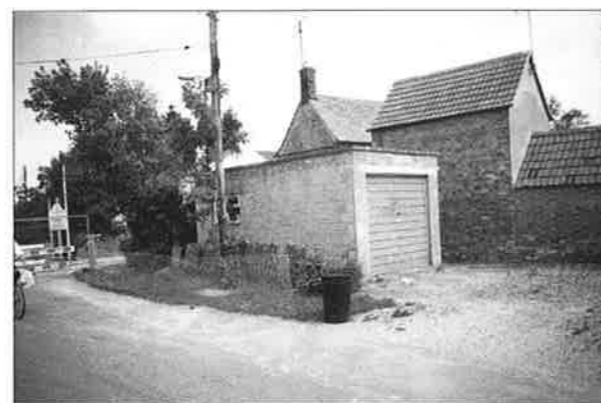
Fig 8: The garage of No.27 is also a poor construction: a flat-roofed rectangle, separated from the road by a line of broken plank-stones
